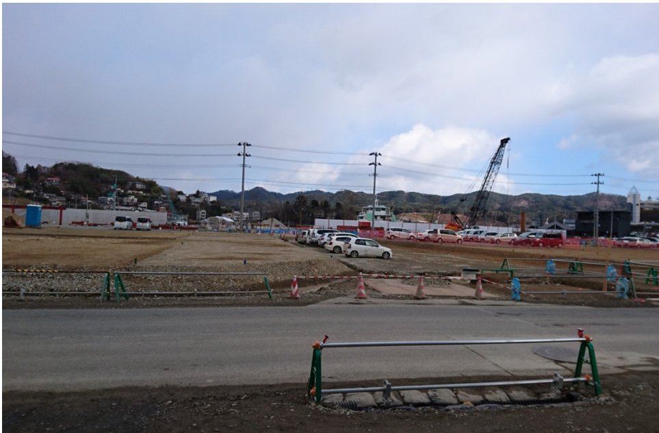
Figure 4. Construction site in the Bay Area in 2017.
